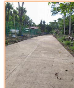
Concreting of Local Access Road, Brgy. Calaran (2020)
