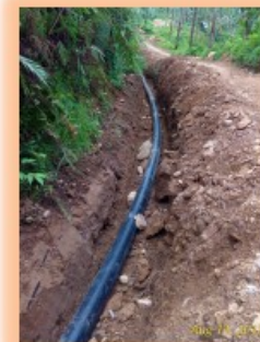
Construction of Calamba Water System Level II and III (2018)
