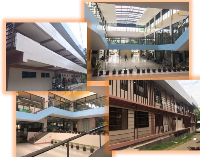
Construction of Calamba Municipal Building (2017)
