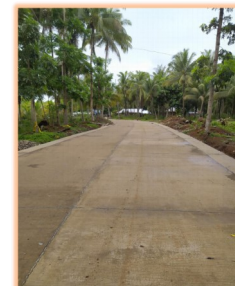
Concreting of Core Local Road in Bunawan Crossing Dapacan Bajo
