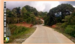
Concreting of Siloy Upper Dioyo Concepcion Road (2014)
