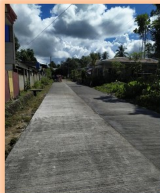
Concreting of Rebosura Street, Brgy. Northern Poblacion (2020)
