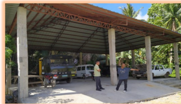
Construction of Residual Containment Area (2019)
