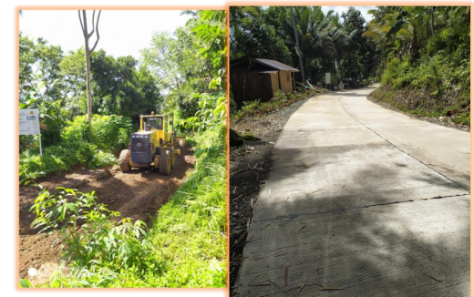
Concreting of Siloy to Mamalad Road (2020)
