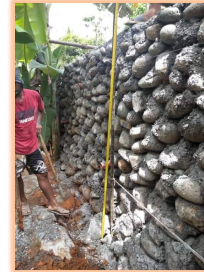
Construction of Slope Protection at Mamalad (2020)
