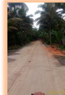
Construction of Sulipat to San Isidro Farm to Market Road (2018)
